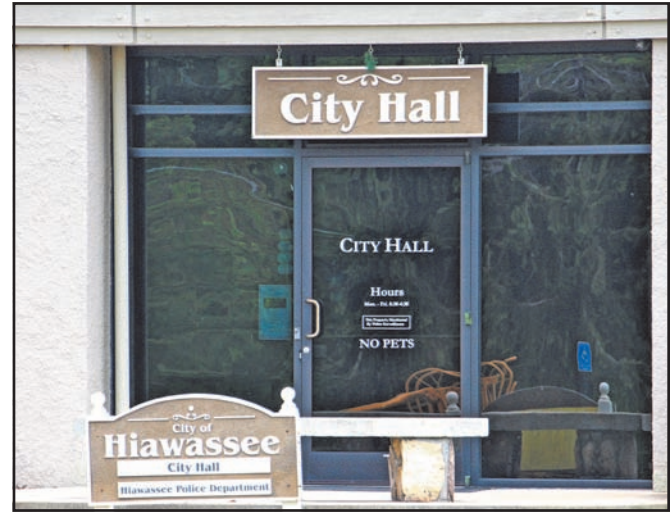
Hiawassee City Hall
